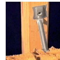
In light frame construction this can become a real problem especially on lower courses with semi cured mortar
